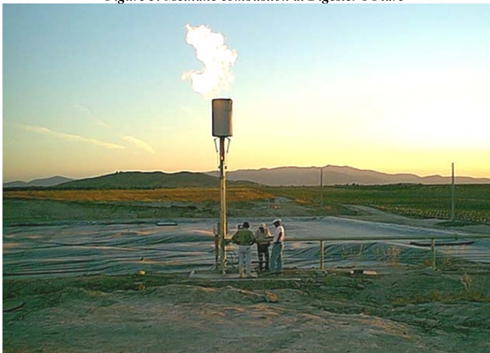
Figure 3: Methane combustion at Digester’s Flare
