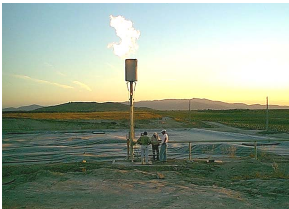
Figure 3: Methane combustion at Flare in Peralillo
